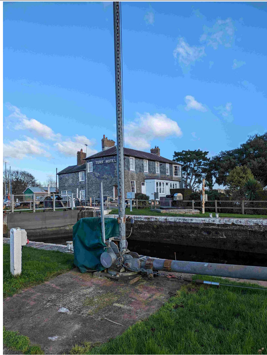
Image B19. Turf Lock Masting Derrick
